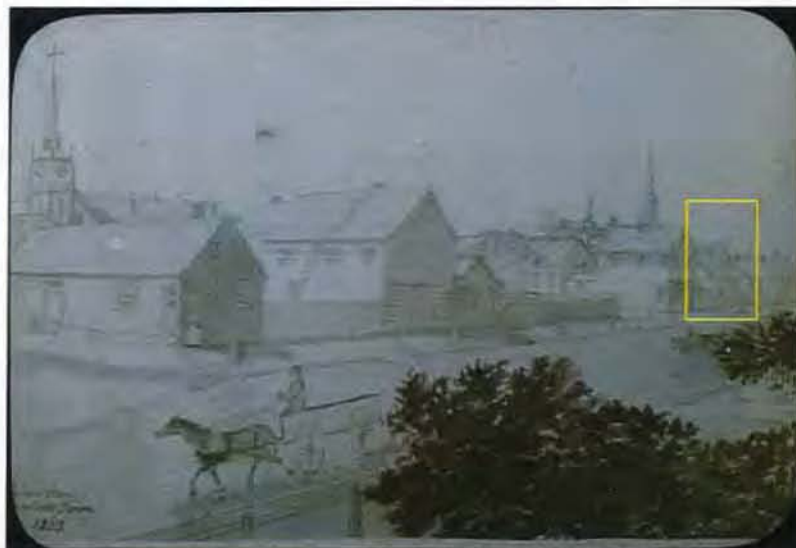
Figure 6. Sketch entitled "Prince Street, Charlotte Town, 1863" from Public Archives and Records Office, Prince Edward Island Acc2702/s23/55) showing the West side of Prince Street as viewed from Water Street. 41 Prince Street shown as a 1 ½ storey house with a small single dormer at the front.
