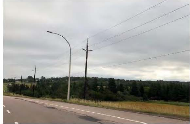
2- VIEW OF SITE FROM BY-PASS HIGHWAY– LOOKING SOUTH-EAST
