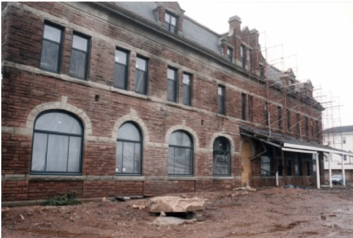
East elevation after window installation in 1996
