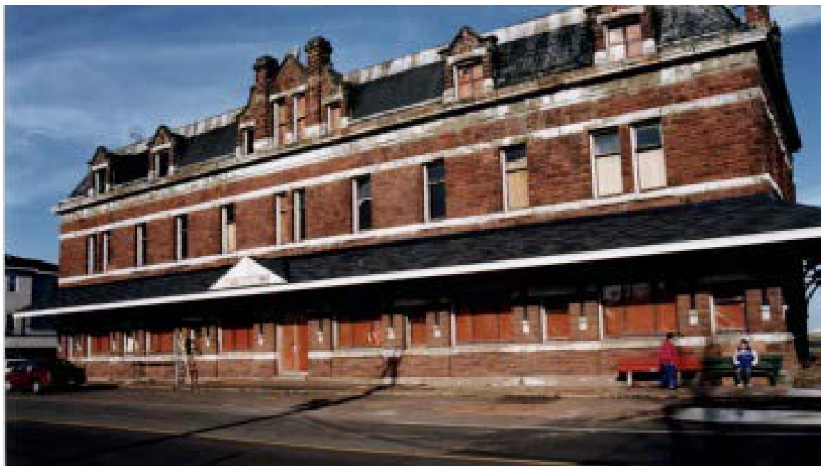
Photo of west elevation prior to 1996 renovations
