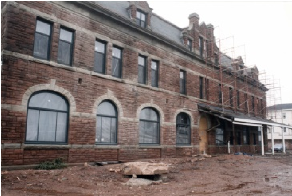
East elevation after window installation in 1996
