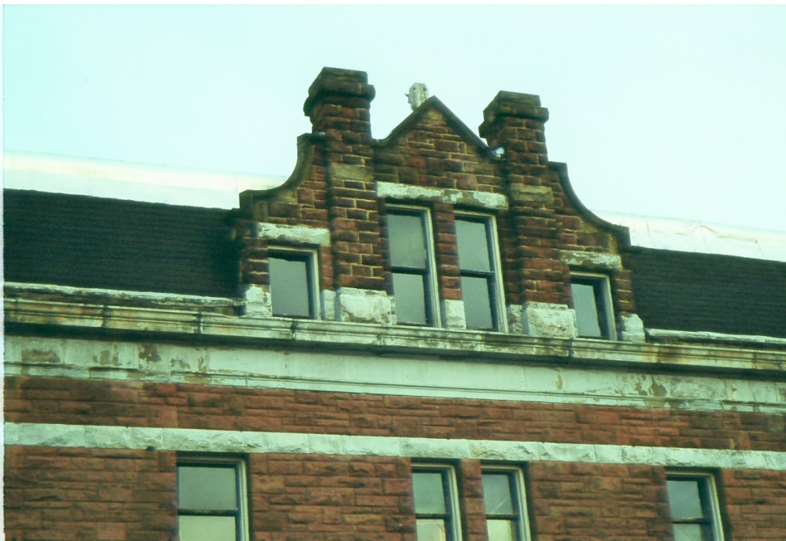
Third Floor window detail c. 1996
