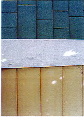
Materiality of Neighboring House
