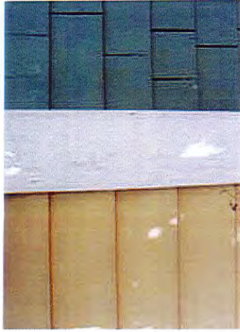
Materiality of Neighboring House
