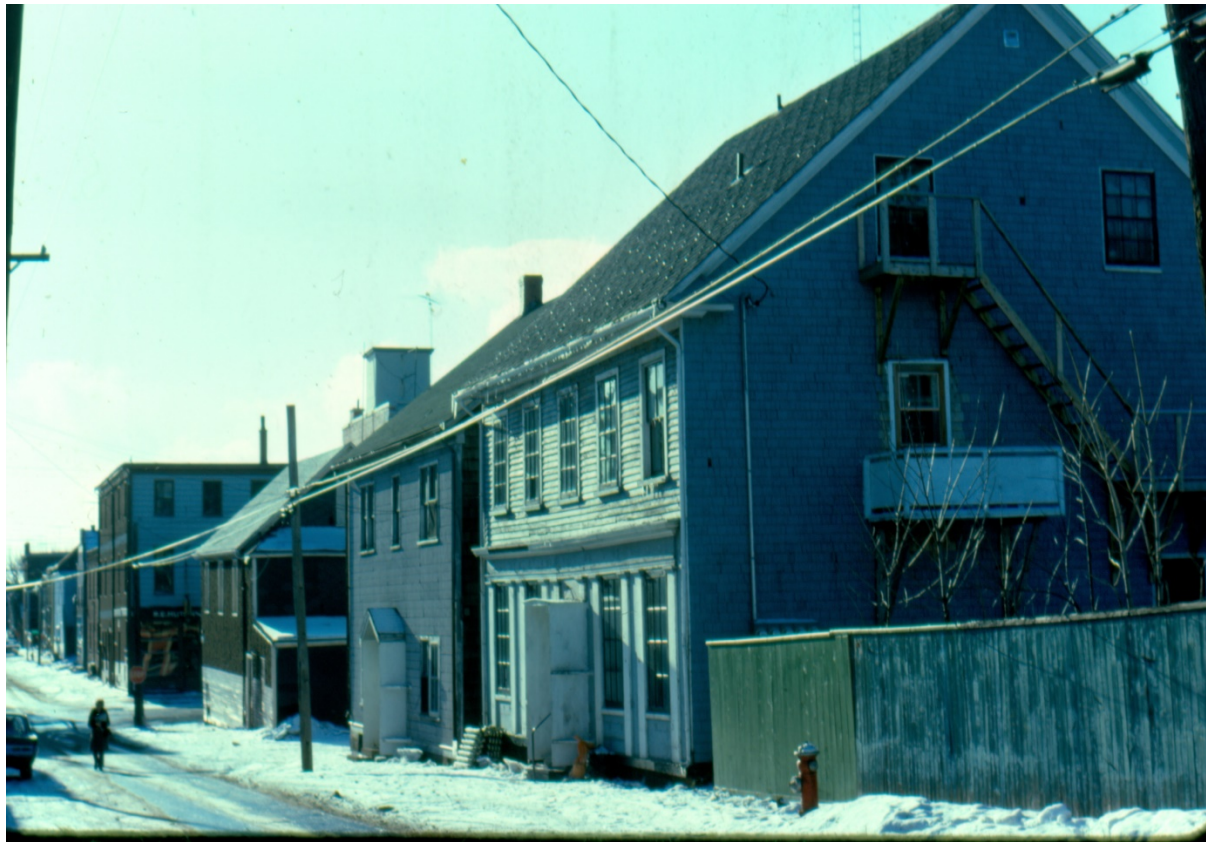
93 King Street & 91 King Street from east side
